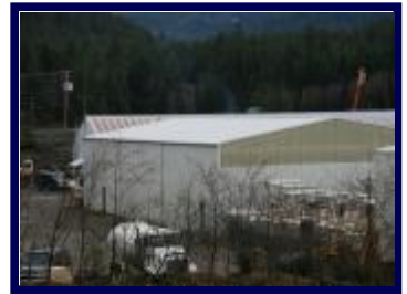
VIEW OF THE BACK OF THE BUILDING
